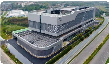
Regional Energy Station in Chengdu Tianfu International Airport New City Area
