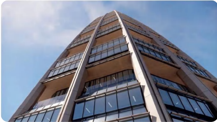
Curtain Wall of Sinochem Holdings Building in Xiong'an
